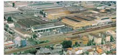
Bolzano plant, Italy (Total surface: 197.049 m 2 )
