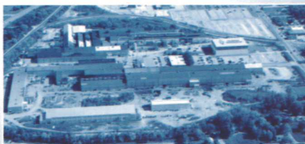
Fort Wayne plant, IN-USA
