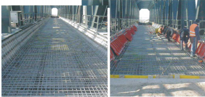
RAIL VIADUCT VENEZIA - PADOVA ITALY
