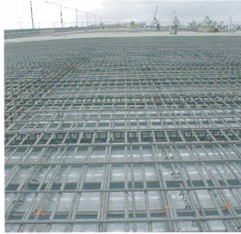
DRISCOLL BRIDGE ON THE GARDEN STATE PARKWAY WOODBRIIDGE, NJ - USA
