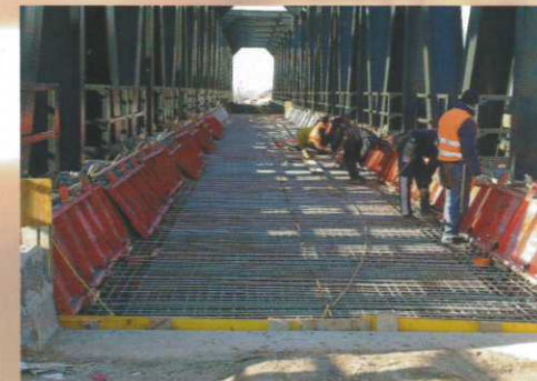
Rail Viaduct Venezia-Padova, Italy
