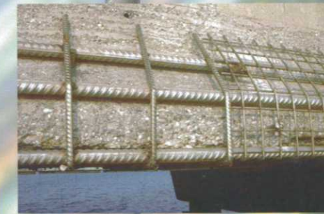
Aleghero's Bridge - Italy
