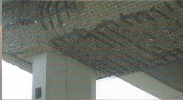
Villastellone Viaduct - Italy
