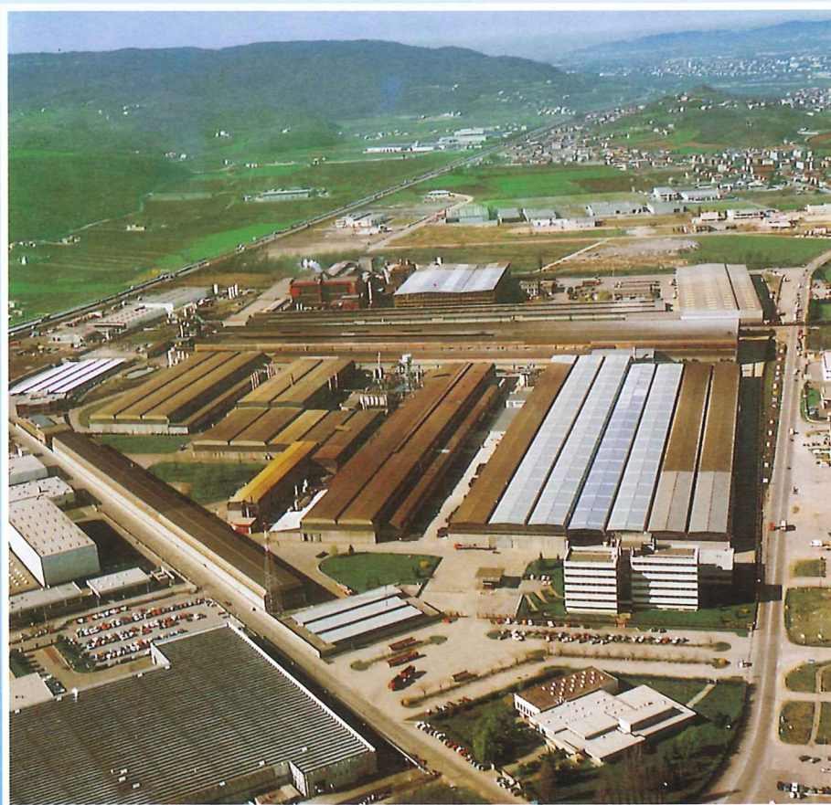
Aerial view of the Vicenza plant
