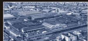
Bolzano plant, Italy
